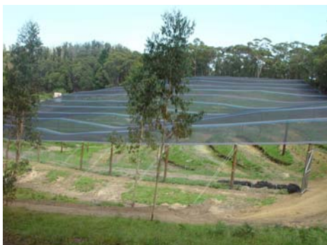
THE SUCCESSFUL STRUCTURE - A JOB WELL DONE !!!
