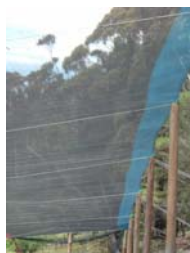
Erecting the net panel by panel.
