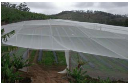
Neville Dhillon's permanent structures erected himself with the help of friends and co-workers.
